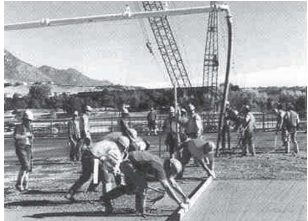
Finishing Concrete Flatwork
